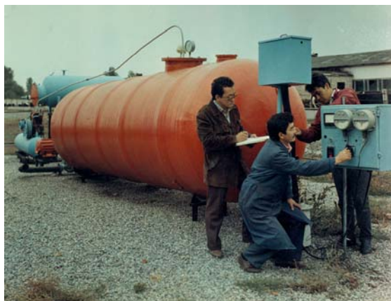
Pic. Fragment test biogas plant
